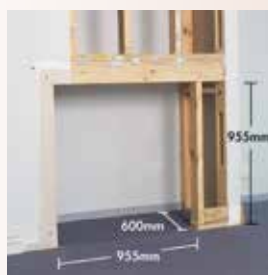
Timber framework partially clad with 12mm Villa Board
